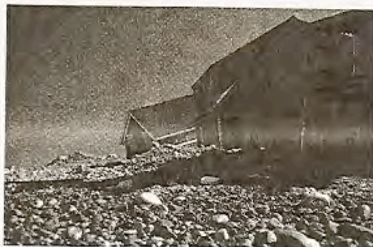
Fig. 5.14 View of houses destroyed in Scituate, Massachusetts, during the Blizzard of 1978. Storm waves and the onshore movement of gravel toppled foundations, leading to the collapse of numerous houses along this section of coast.
